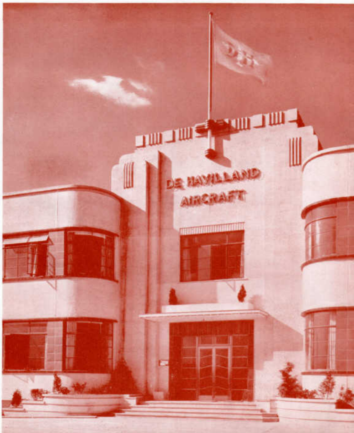
The entrance to the office building of the de Havilland establishment at Hatfield.
