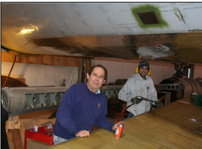
Steve Belanke and Mike King repairing elevator corrosion
