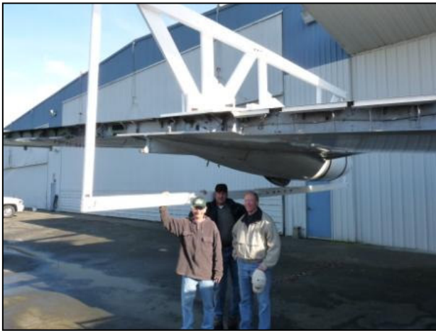
Figure 2 Pannier Tank Cable Support Beams
