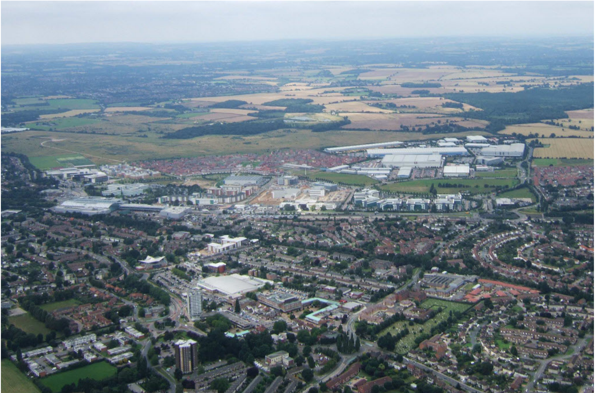
Looking north-west. The Police Station, formerly the Administration and Canteen blocks, is in the centre.
