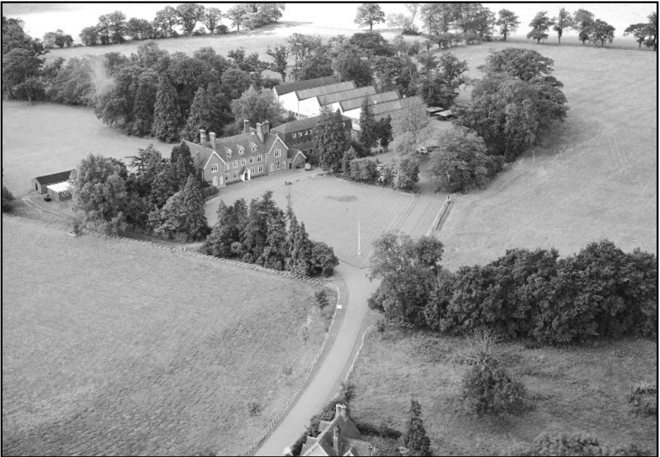
Astwick Manor, hostel and workshop, 21st August 1957
