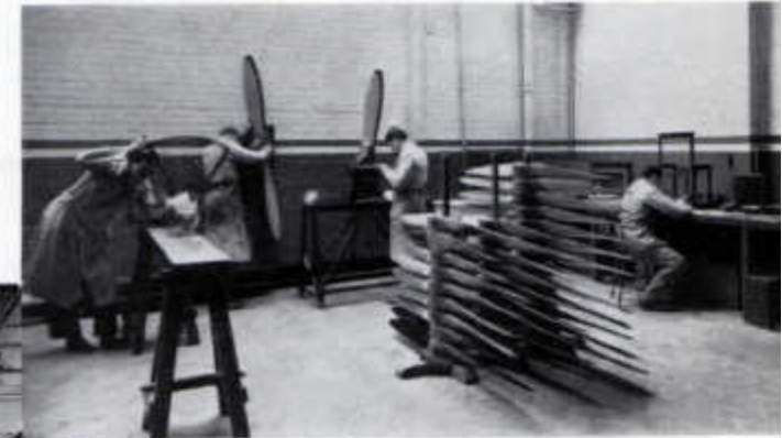
In the upper picture, students are shown checking balance and pitch of wooden air screws and finding the moisture content of timbers.
