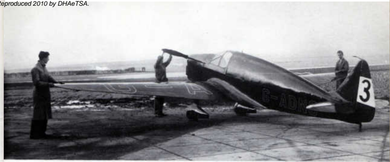
T.K.2. A high-performance single-seater designed and built entirely by de Havilland students. This aeroplane was placed fourth in 1935 and sixth in 1936 in the King's Cup Air Race. It also won the Heston to Cardiff Air Race in 1936 at an average speed of 189.2 m.p.h.
