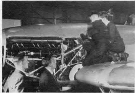
Instruction on Hurricane overhaul and repair.
