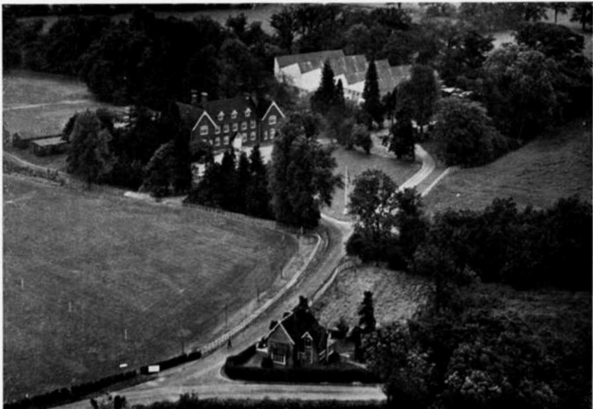
Astwick Manor, Hertfordshire, the headquarters of the School.
