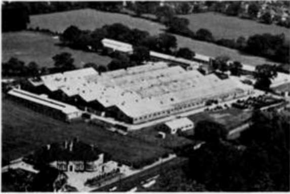
A jet-engine factory at Edgware.
