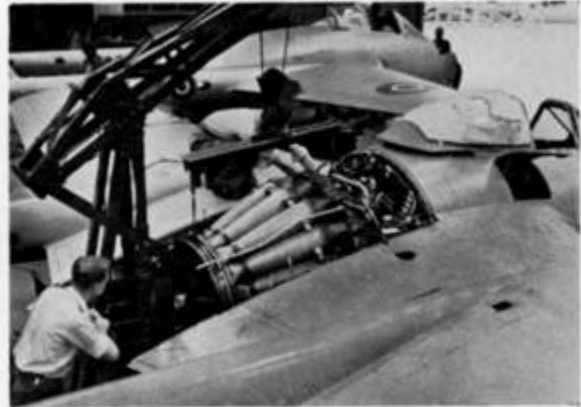
Apprentices fitting a Goblin engine in a Vampire.
