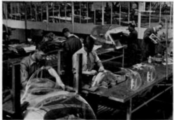
Work on plastic canopies.
