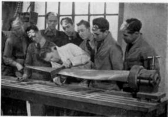
1935. Learning the new technique of propeller production.
