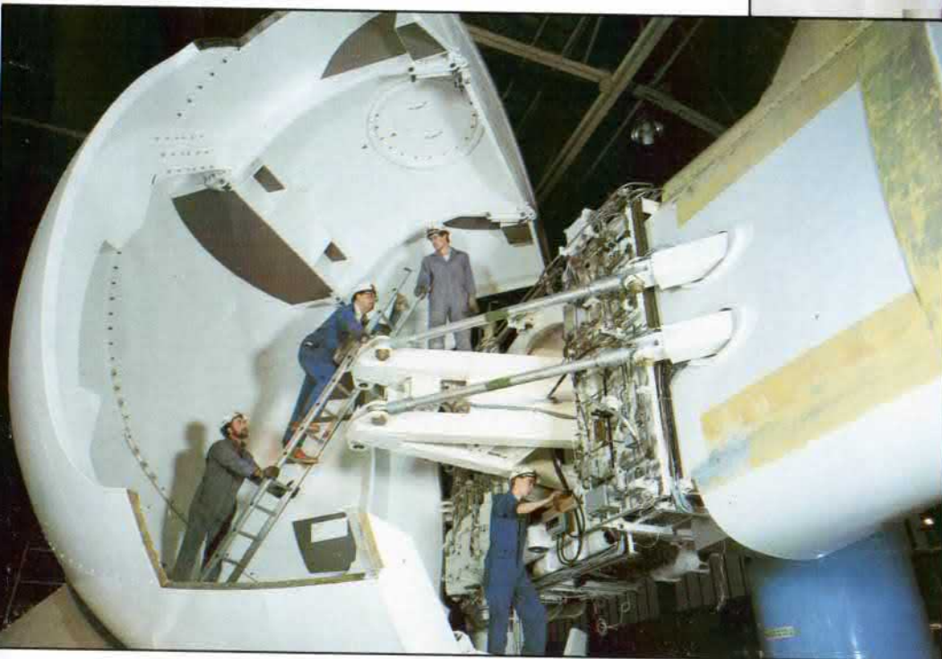
Working inside the spinner of the 60 metre diameter turbine rotor.
