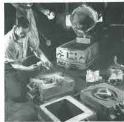
The oil sump shown being cast in magnesium alloy is supplied by J. Stone & Company (Charlton) Ltd.
