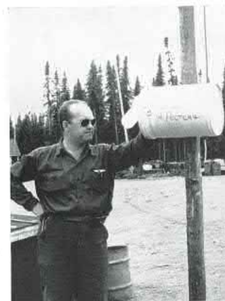
Are you there? Time-saving devices are utilised by Fecteau Air Transport to speed up the movement of traffic at the Company's fixed air bases. Valere Guay, Base Manager at Cache Lake, carries on two-way conversation over loud-speaker installation at the seaplane dock with the base office. Many such installations help direct the handling, loading and despatch of the Company's aircraft.
