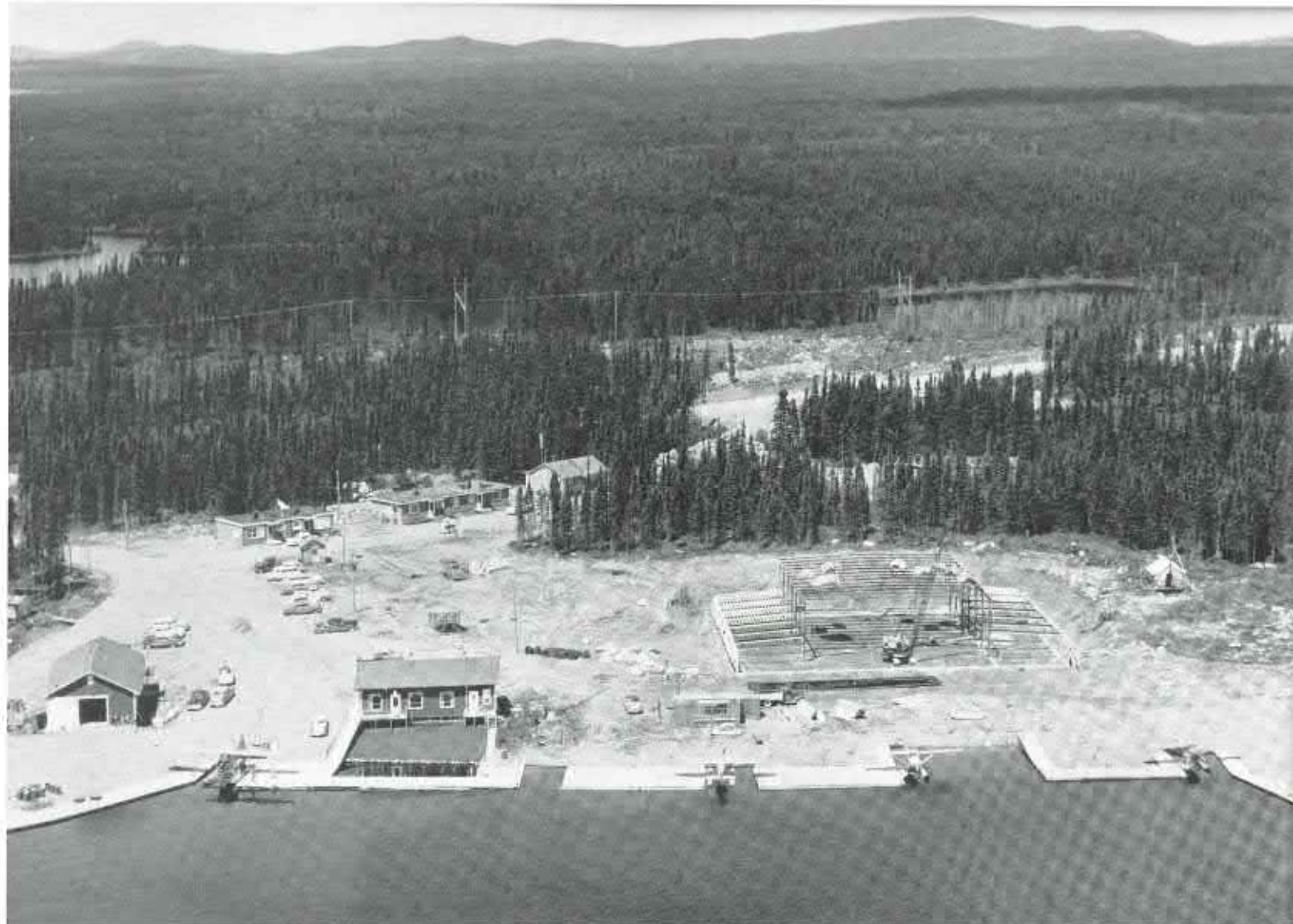
New voices in the Wilderness. Fecteau airbase at Cache Lake in the heart of Quebec's newest copper-mining country, Chibougamau. Dock is 1,200 feet long, accommodates 17 seaplanes. New steel and concrete hangar (right foreground) is under construction at cost of $130,000. Start on housing project for company personnel may be seen at upper centre. Site was untrodden virgin forest four years ago.
