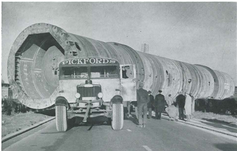
From the outset the Gyron Gynorm was developed for operation with reheat. An early version of the afterburner assembly is here seen on its journey from the Engineering Division at Stag Lane to the test bed at Leavesden. Subsequent development work enabled some reduction to be made on the weight of this interesting component.
