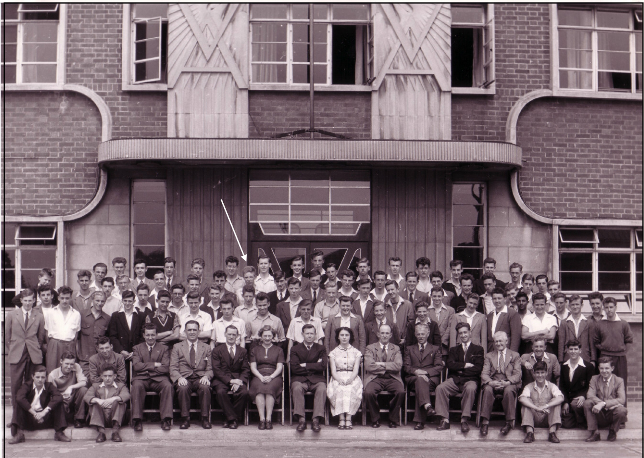
The main entrance to de Havilland, Chester and the 1954 intake. The factory was built by Vickers-Armstrong just before WW2, hence the VA letters on the pillars.
