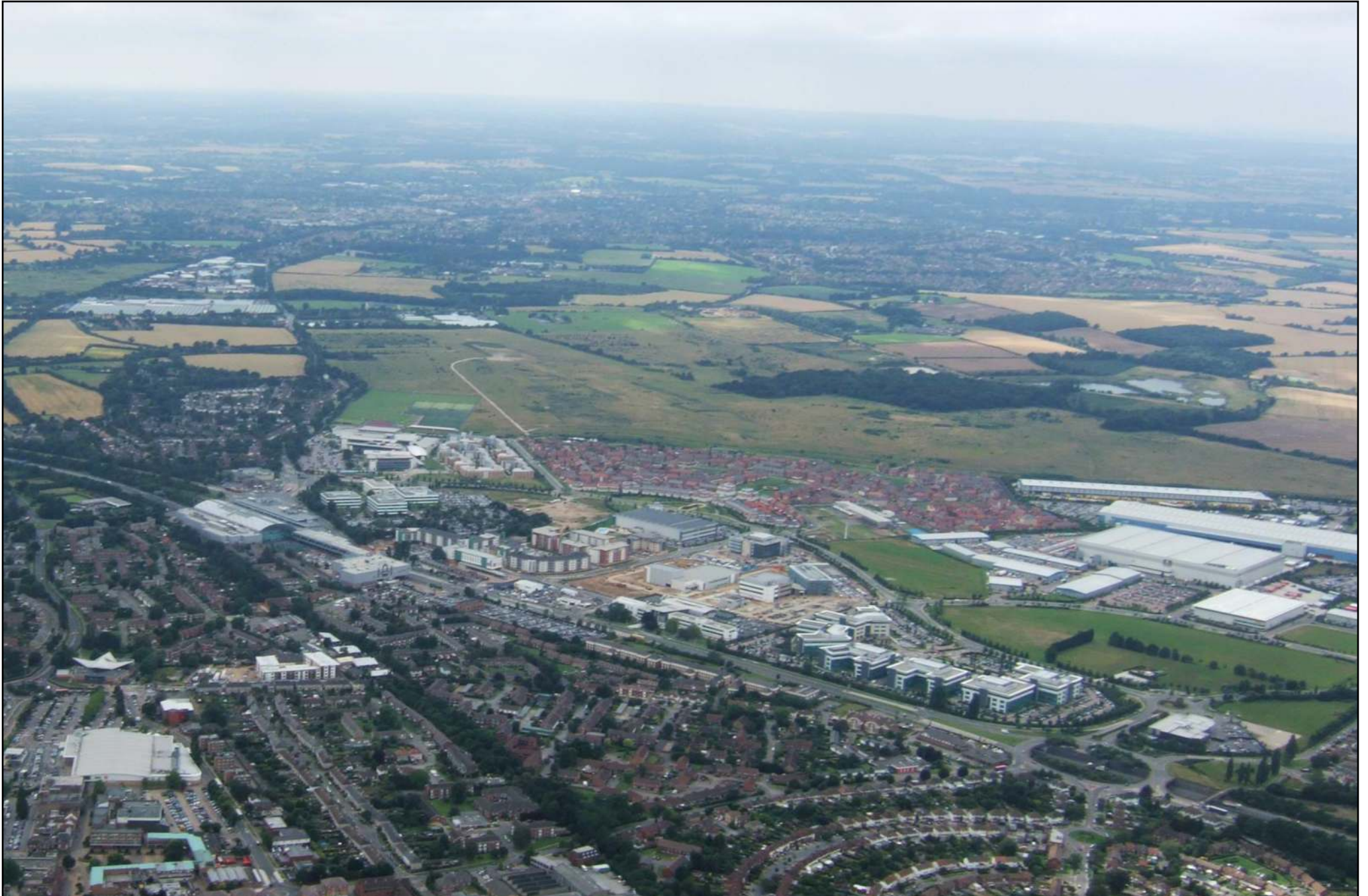
22nd July 2008: looking towards St Albans. Building work is in progress in the centre, on the site of the main factory area from the 1940s onwards.
