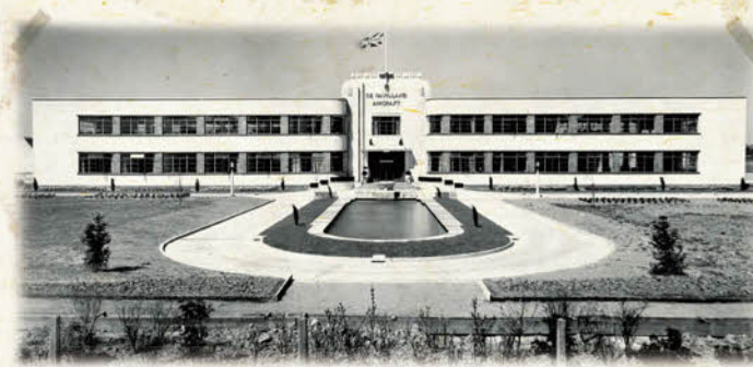
Front entrance of the Administration Block. Courtesy of BAE systems
