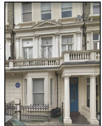
32 Barons Court Road. Google Street View Nov. 2017. The building has four storeys. In his autobiography Sir Geoffrey refers to "our flat".
