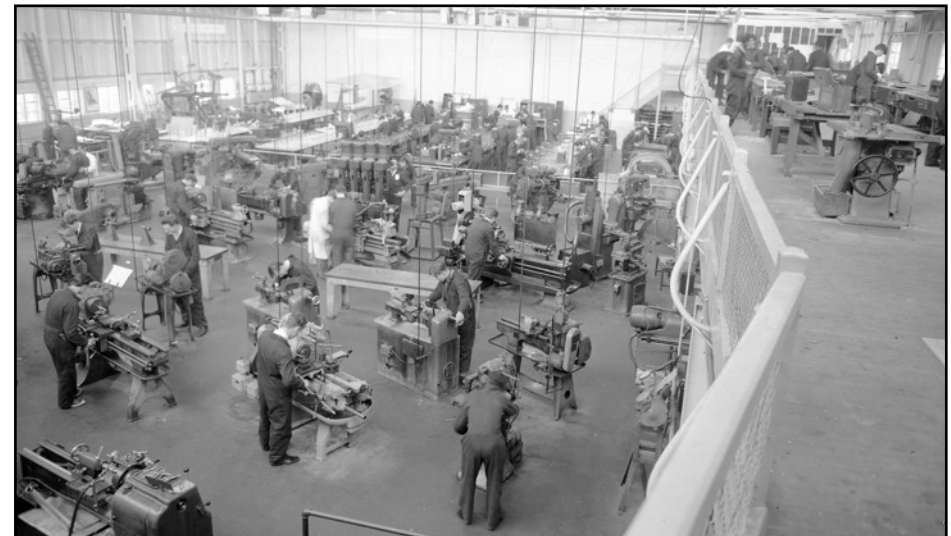
Astwick Manor workshop, December 1963. Woodwork section on balcony at right.
