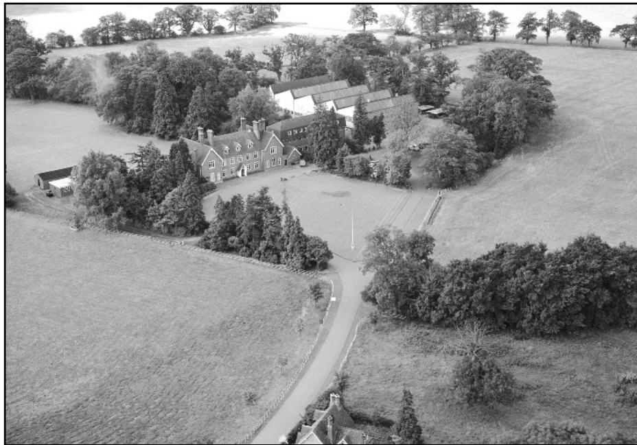
Astwick Manor, hostel and workshop, 21st August 1957
