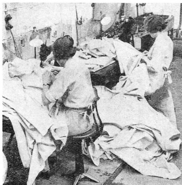
Many thousands of yards of the finest Irish linen are used for the coverings of wings and other surfaces in a big aeroplane factory in the course of a year. On the left fabric is being prepared for wings, and on the right a tail plane is being covered.
