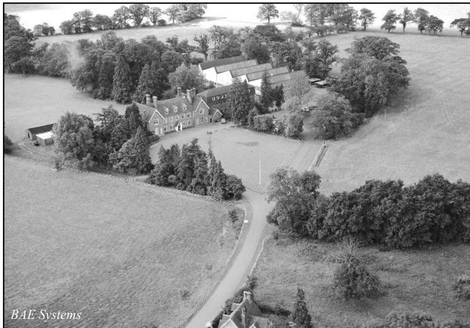
Astwick Manor, hostel and workshop, 21st August 1957
