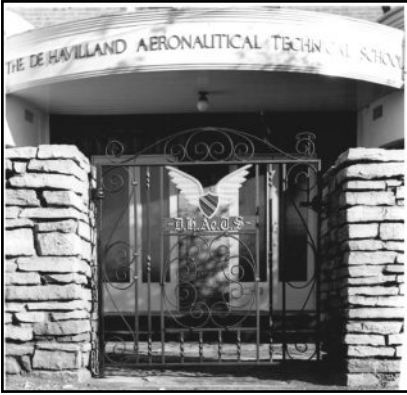
Entrance to DHAeTS Christchurch
