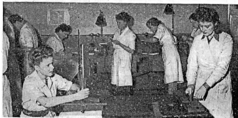
Part of the E. & P. Divn. tool room, women's section. At the table on the left is Miss Betty Gould, marking out a template, and on the right Miss Margaret Shorter is straightening one on the blue surface plate.
