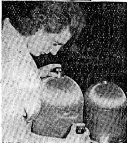
Miss A. E. King, checking concentricity of the hydro-matic dome, and outside dimensions. It was after a short period in a government training centre that she joined the Propeller Divn. in July last as inspector, and is typical of the many girls who are making a good show of an unaccustomed job.
