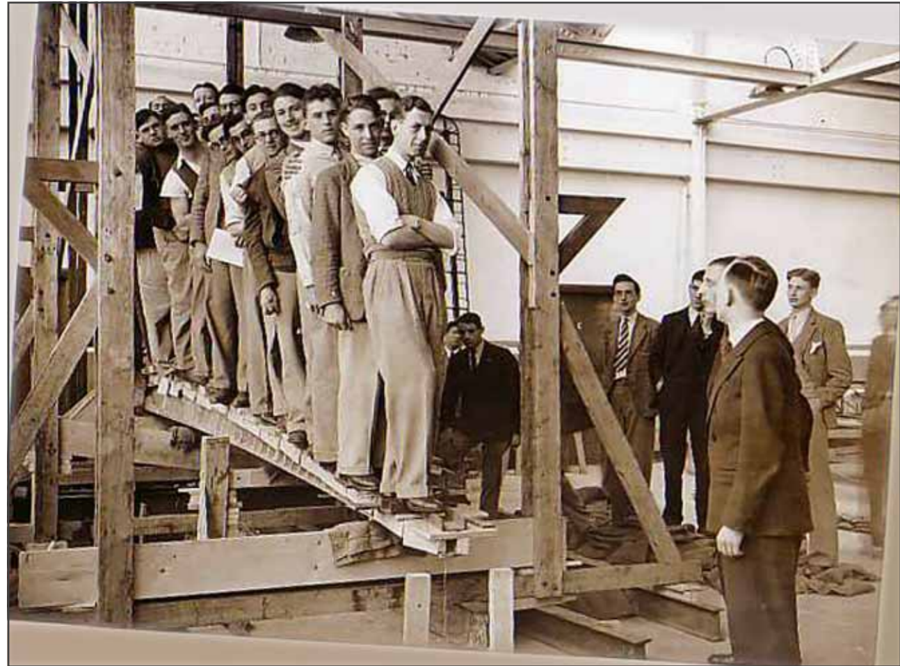
1935 - DHAeTS Students testing the T.K.2 wing. Photograph found on the internet by Ted Lawrence (1957-62), straightened and enhanced by the compiler. See also Page 6 of the DHAeTSA Newsletter, Autumn 2008.
