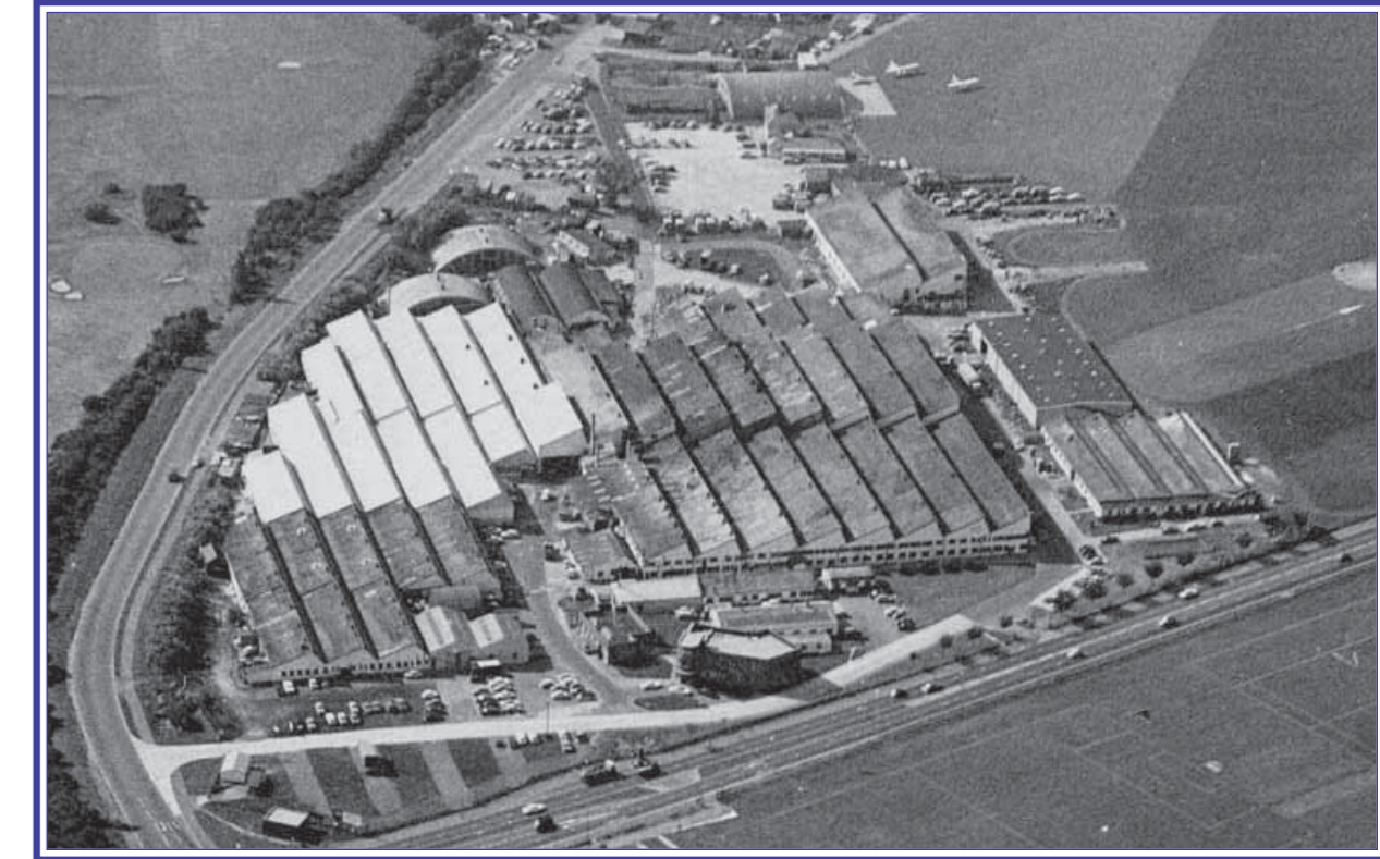
THE PORTSMOUTH FACTORY, HAMPSHIRE.
